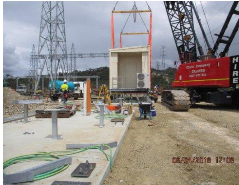
Installation of Powerlink Control Building
