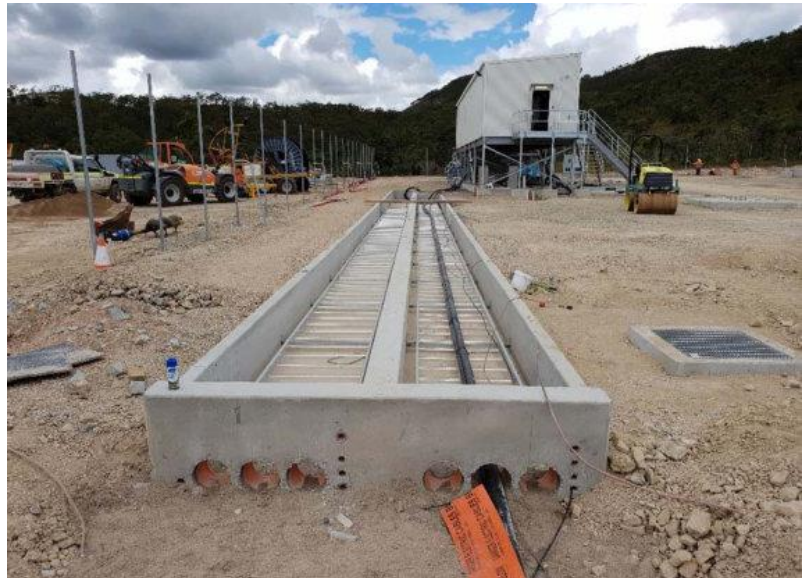
First collector cable placed into substation
