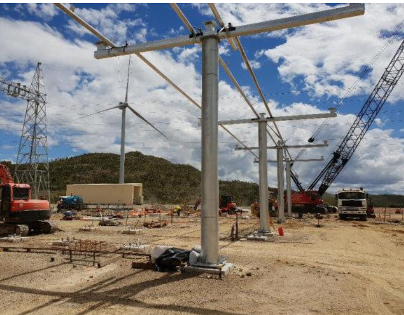
Powerlink switchyard construction works
