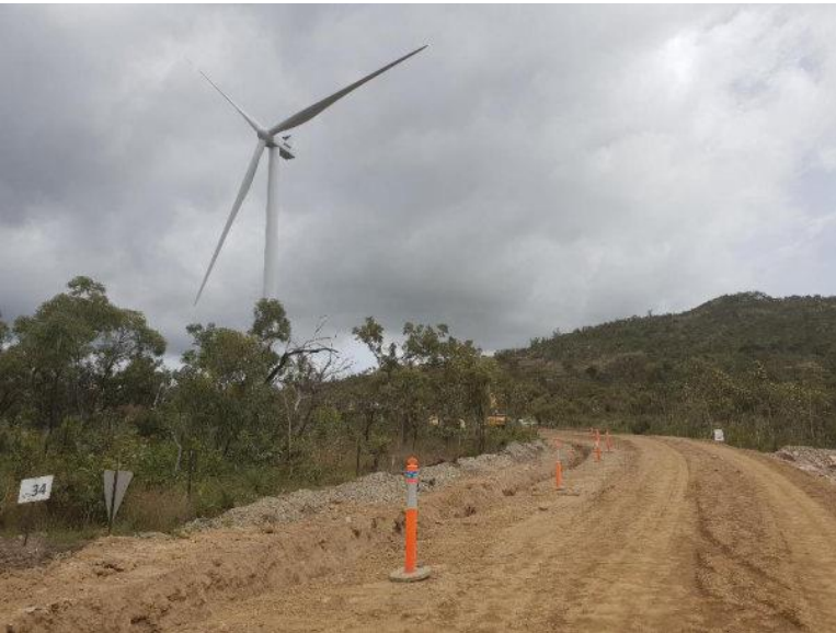
Cable trenching and laying to WTG27
