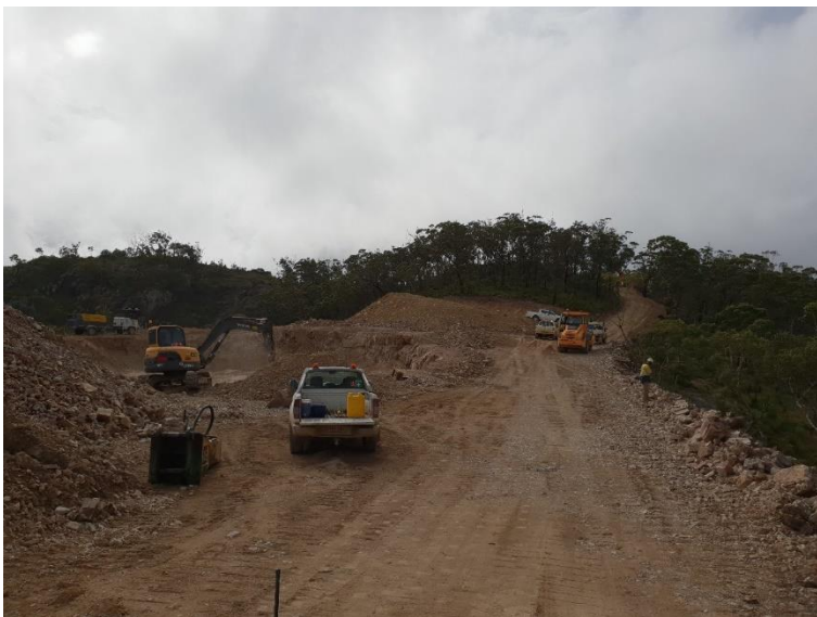
WTG32 - Excavation and access road
