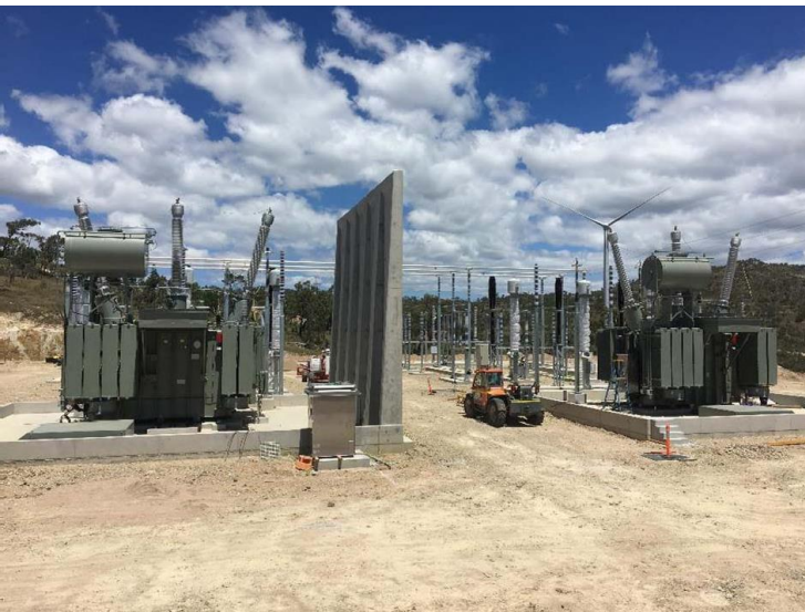
Wind farm substation construction progress
