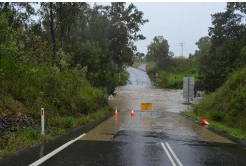
Granite Creek causeway
