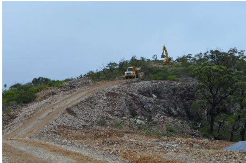
Road construction to WTG 31-32
