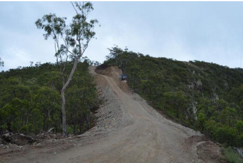
Road construction to WTG19
