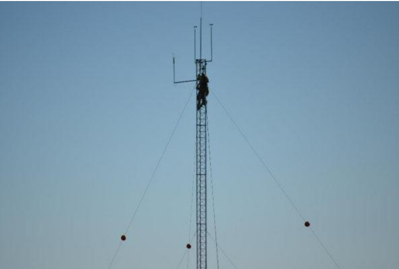
Installation of monitoring equipment
