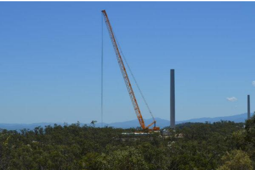
Installation at WTG 45
