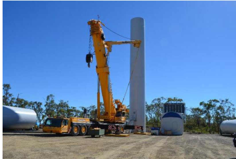
Commencement of installation of WTG 45
