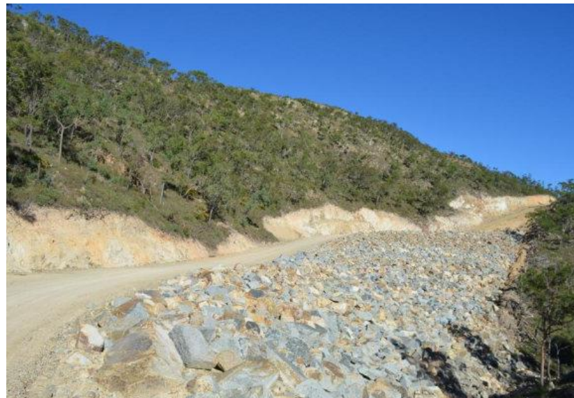
Access Road to WTG 11
