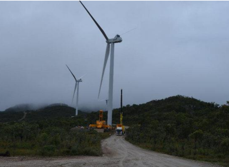
Completion of WTG 36
