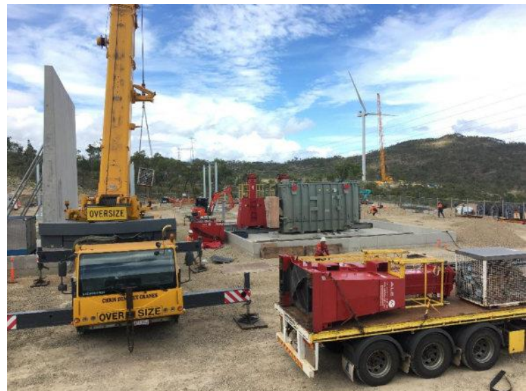
Installation of second main transformer
