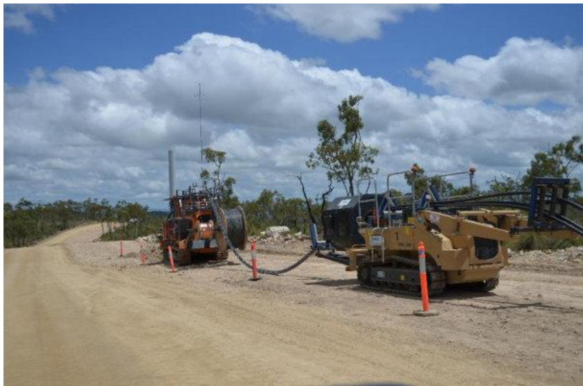
Cable laying between WTG 41 - 43
