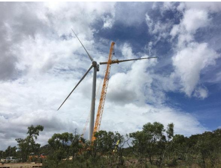
Final blade install at WTG 34
