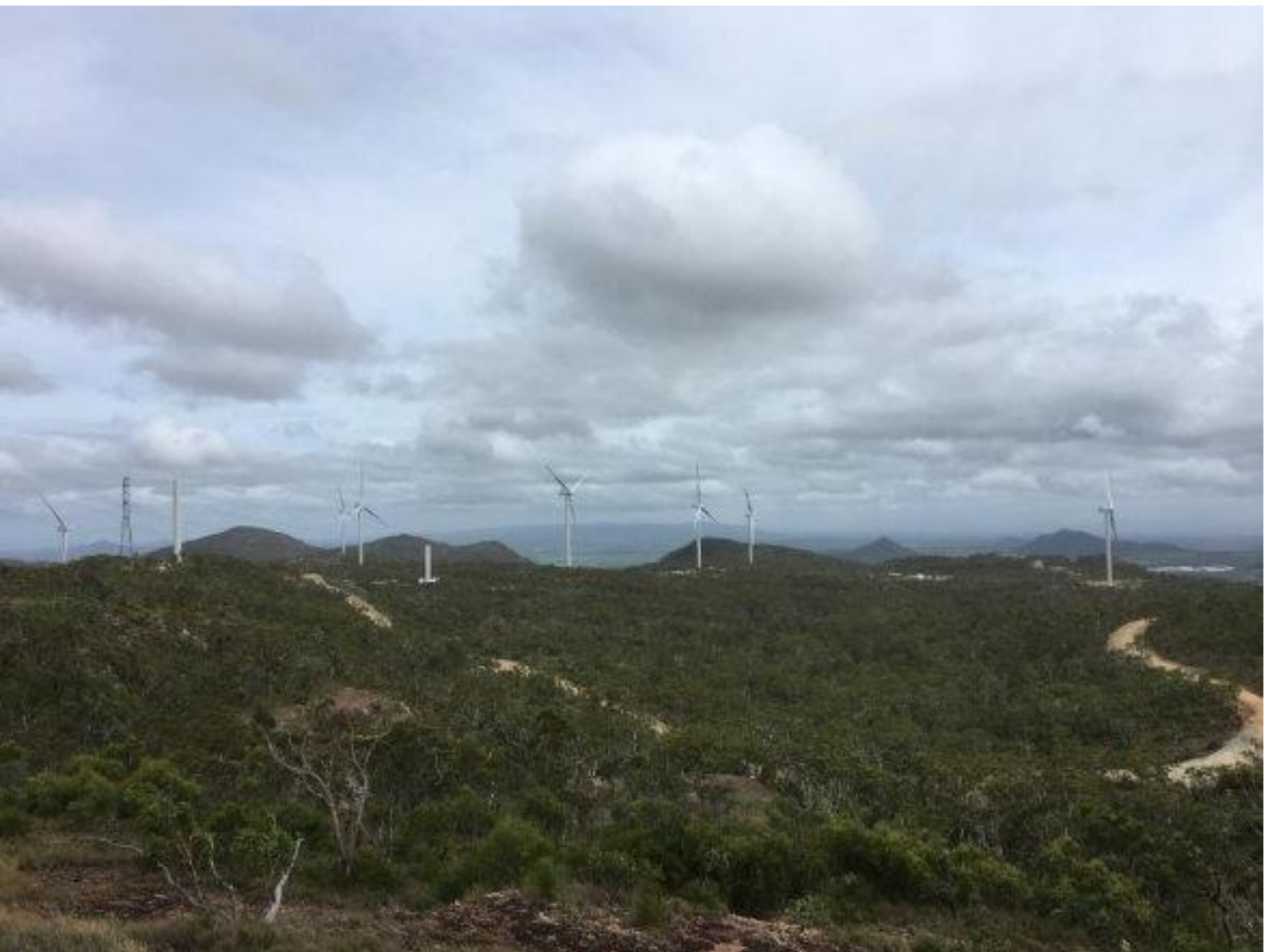
View from WTG 17 looking north towards erected turbines 3 – 9
