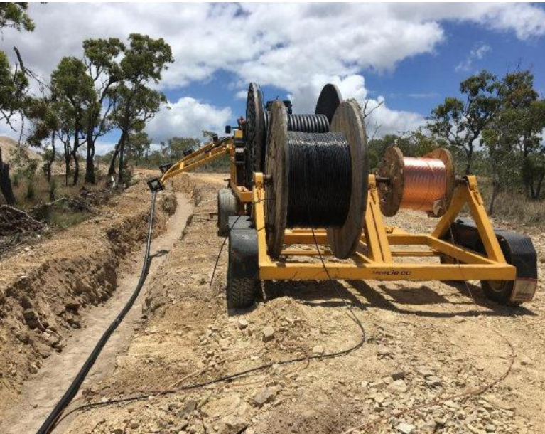
Underground electrical cable laying
