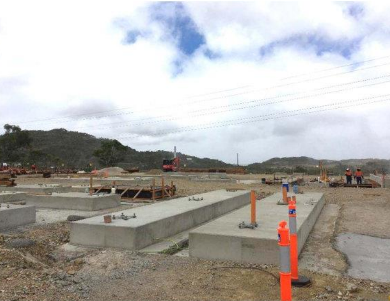
Foundations at wind farm substation
