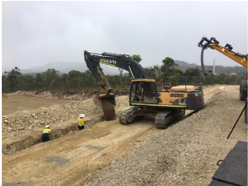
Backfilling of cable trench
