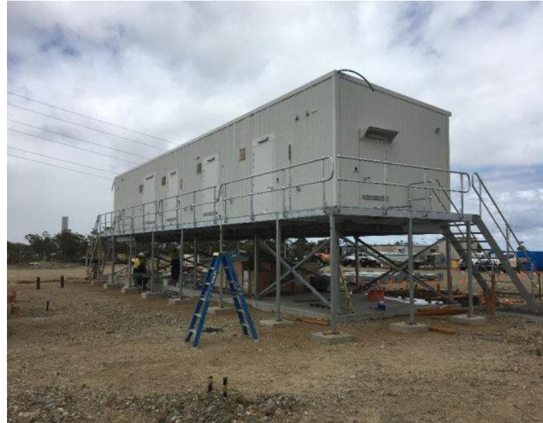
Substation control building
