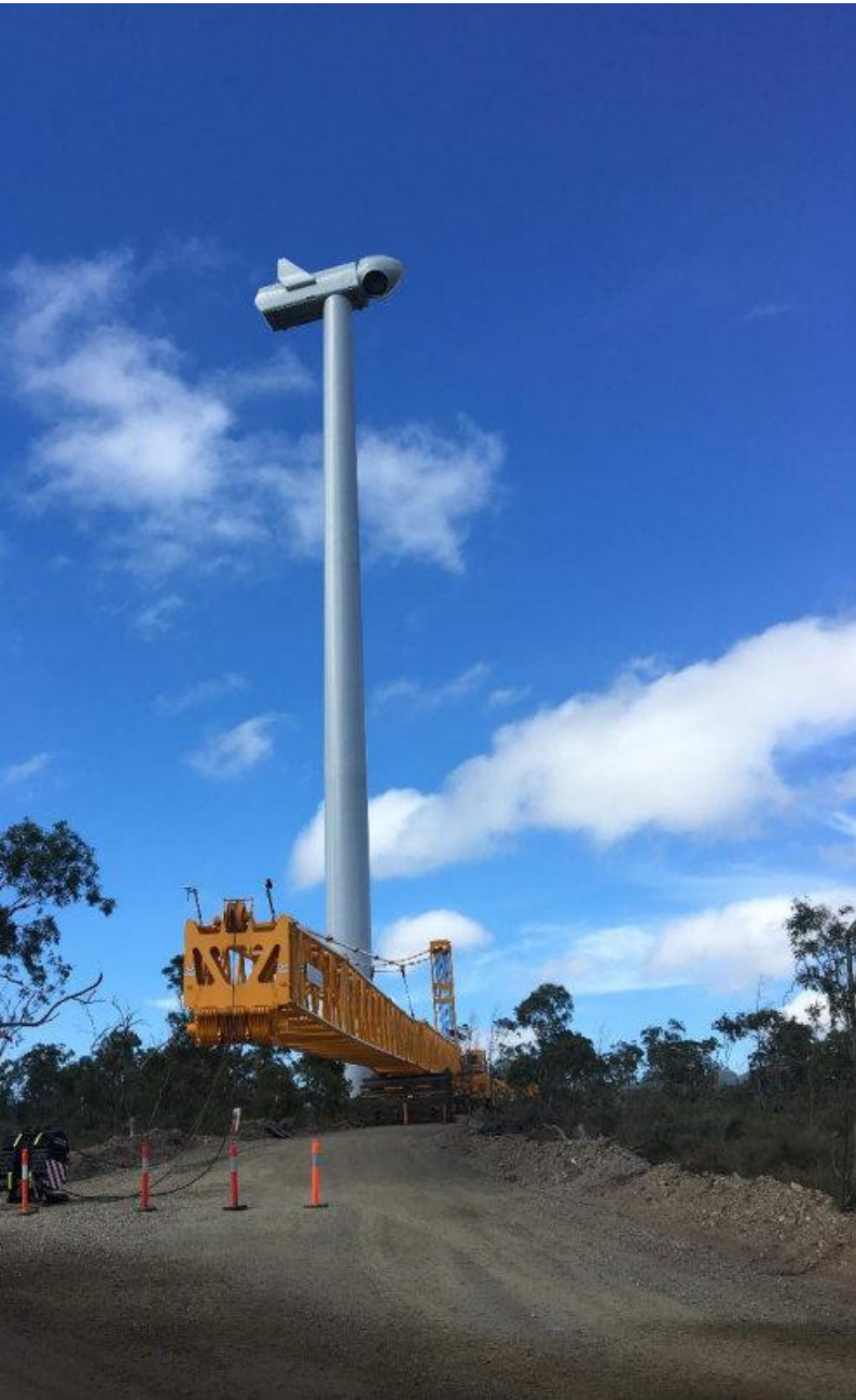
Crane secured for shutdown at partial complete WTG 6
