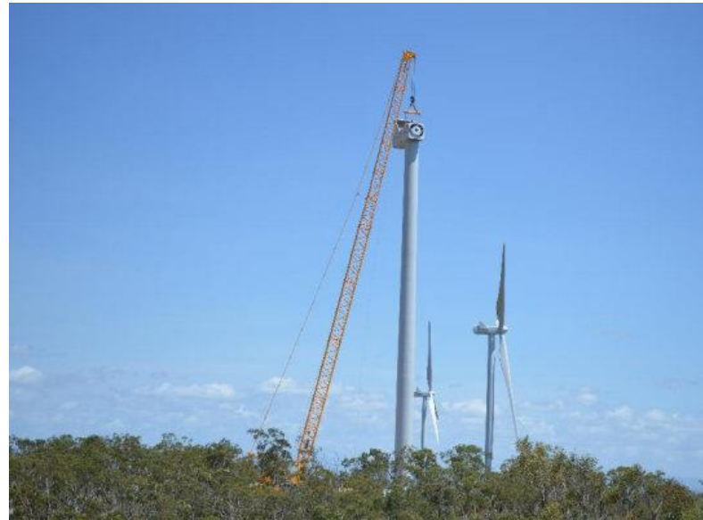
Nacelle install at WTG 6
