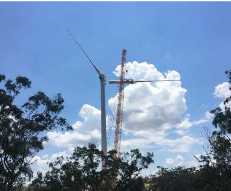
Blade installation at WTG 8
