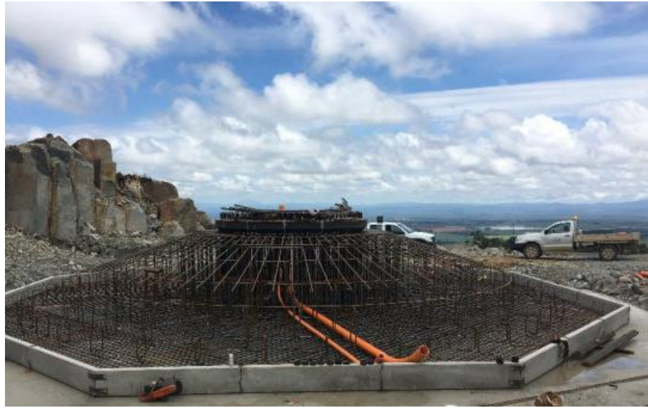
Preparation of WTG 1 Foundation
