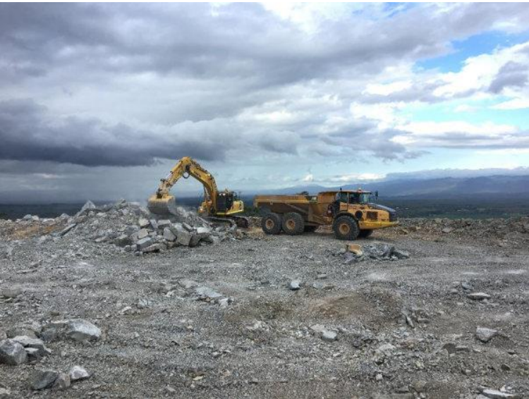
Hardstand excavation at WTG1
