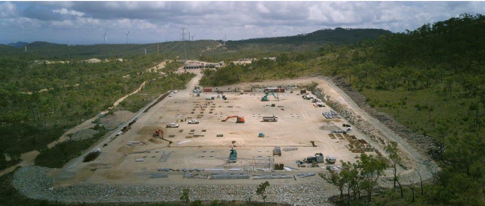
Construction at the Powerlink Switchyard with completed turbines in background
