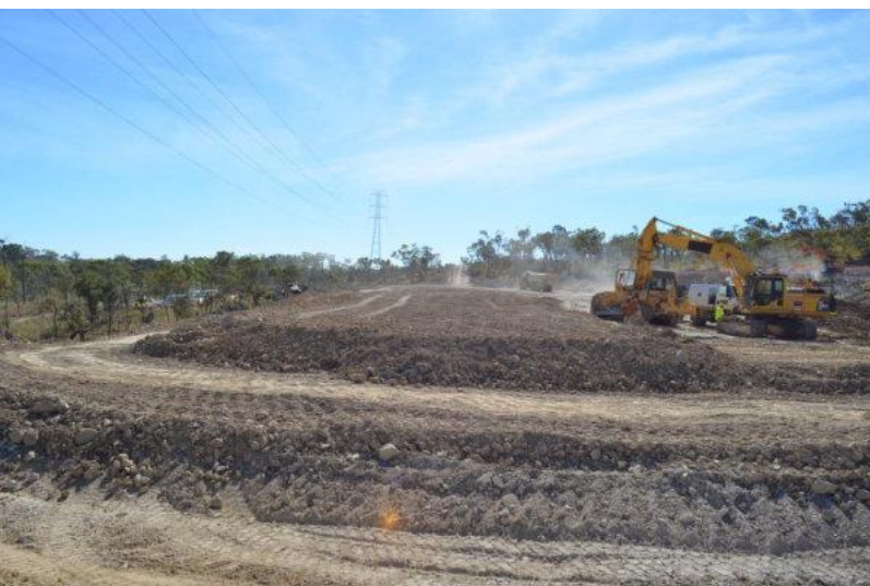
Earthworks at Powerlink Substation Bench
