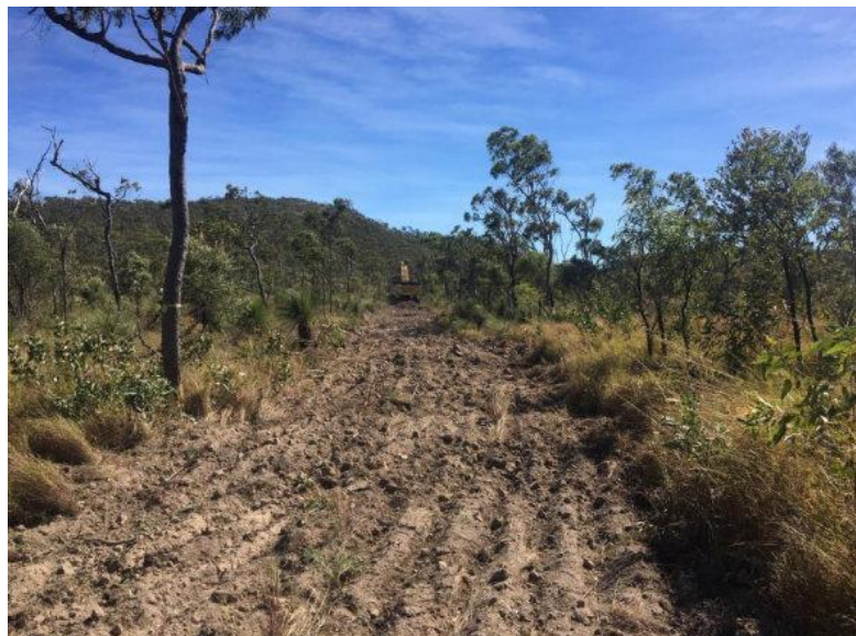
Vegetation Clearing works to WTG 53
