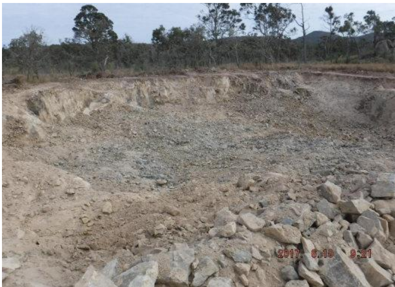
Foundation excavation at WTG #3
