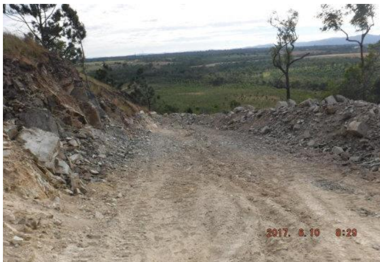
Site Entry Road foundation prep for sub-base
