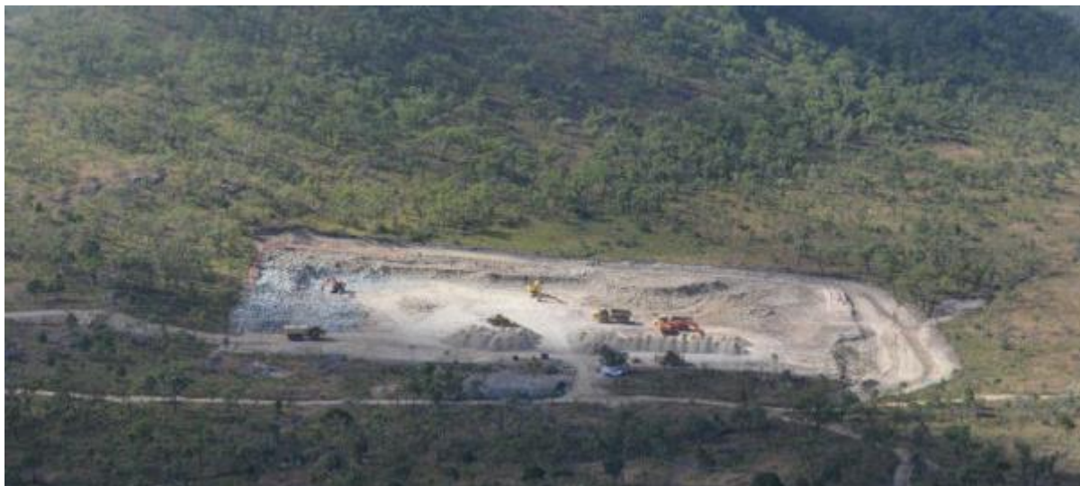
Aerial image of Powerlink bench construction
