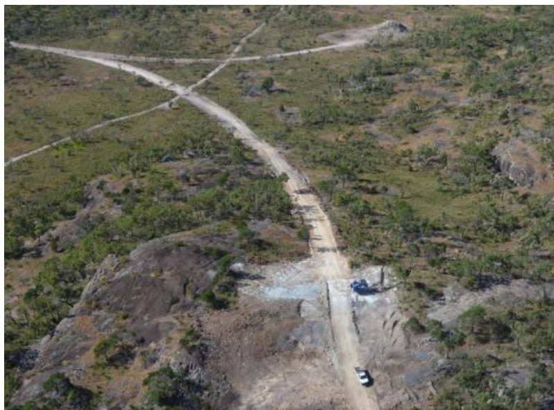
Access Road and hardstand for WTG#35
