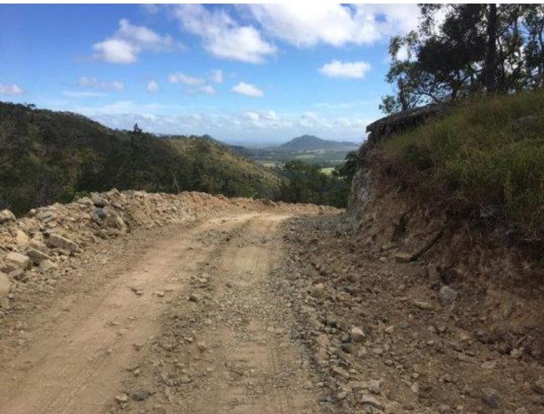
Site Entry Road
