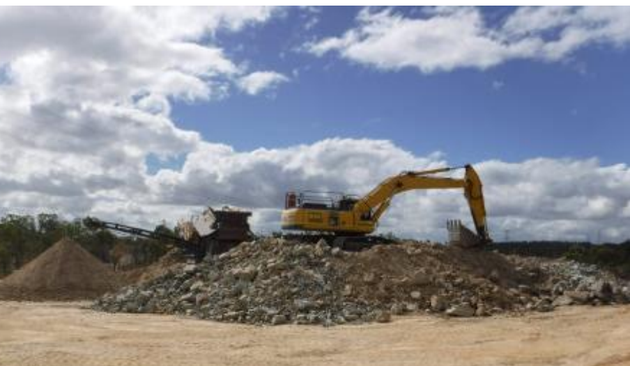
On-site rock crushing and screening
